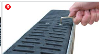
6 Place grating into the channel and tighten the fixing using the security locking key
